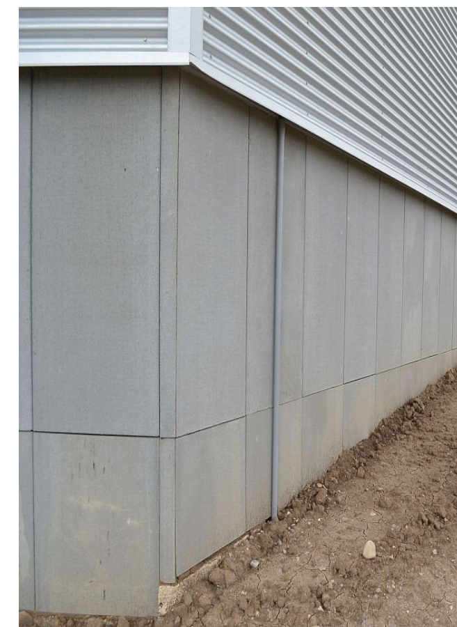
Wallguard - Concrete faced insulated perimeter wall.
